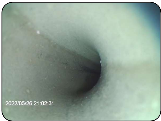
Tube inspection using a Hawkeye Q Video Borescope
